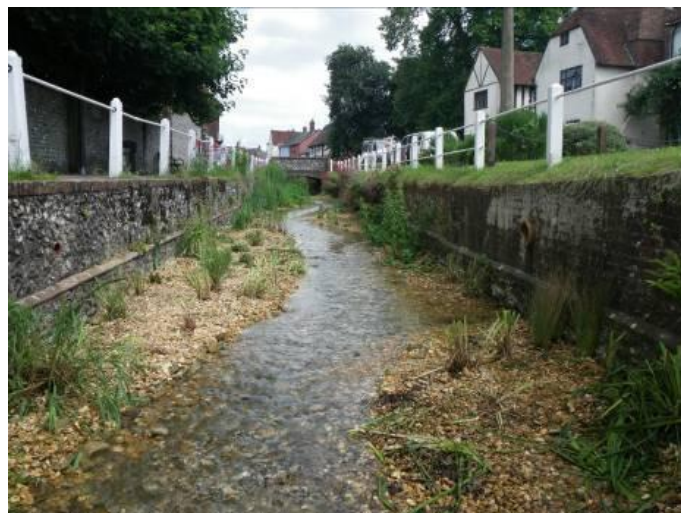
After restoration 'a semi-meandering naturalised channel'
