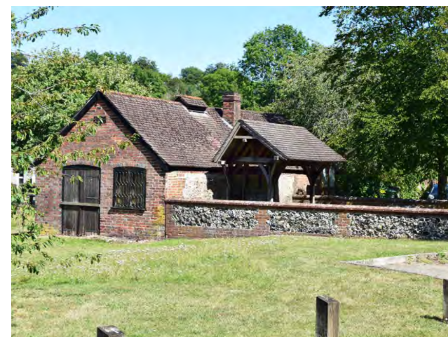
The flint walled enclosure of the historic village Pound, (including a relatively modern shelter) sitting within the green, adjacent to the former Blacksmiths premises.
