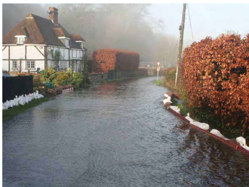
Flooding can occasionally cause severe problems within Finchdean, as seen here on the lane towards Chalton
