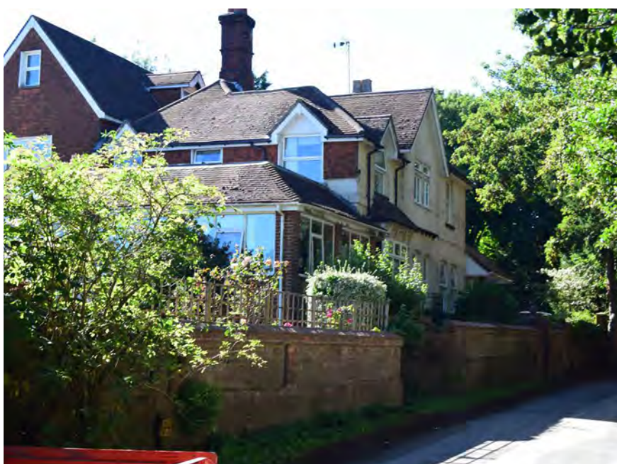
Beechwood House Nursing Home is a large, imposing building on Woodberry Lane, with some building extensions which are unsympathetic to the original architectural style.
