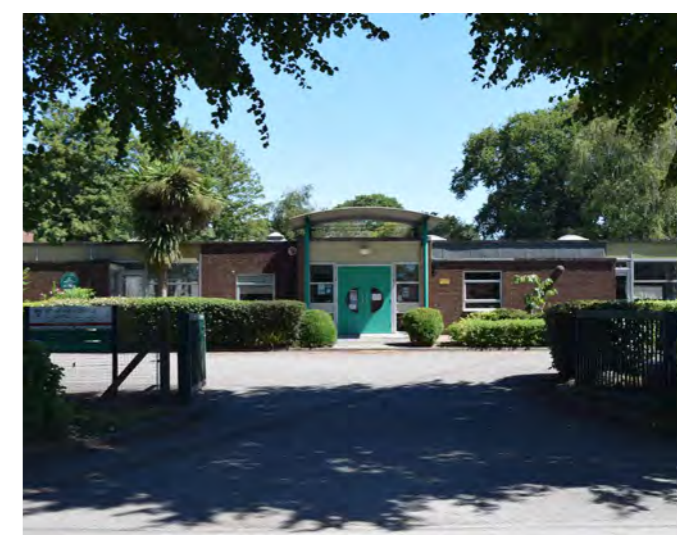
The primary school is a low-level building with a large footprint, set in extensive school grounds, partly asphalt surfaced alongside a playing field surrounded by mature trees.
