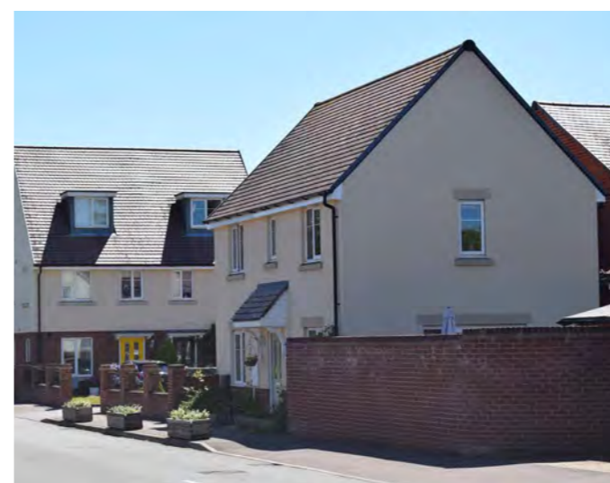
Blank walling of rear gardens siding onto the public realm at Oaklands Avenue.
