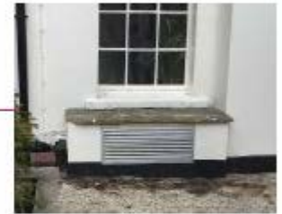
existing low level structures to house proposed AHU supply / extract ductwork
