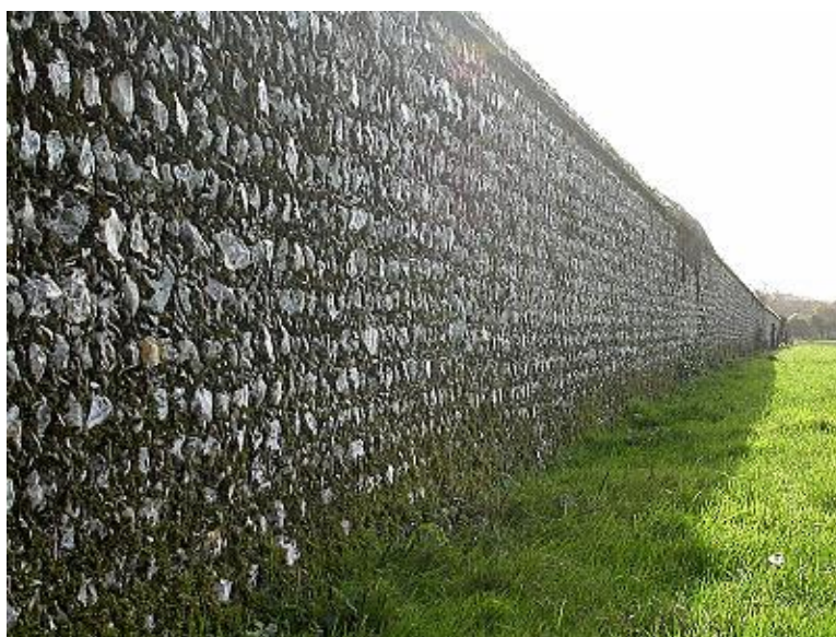
Fig. 5 Flint used in wall construction
