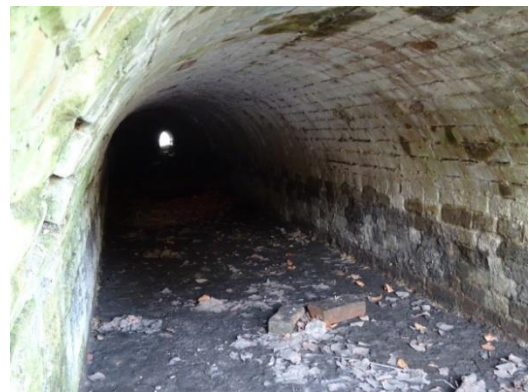
Inside the culvert after clearance
