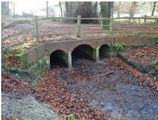
Entrance to the 42 metre long culvert
