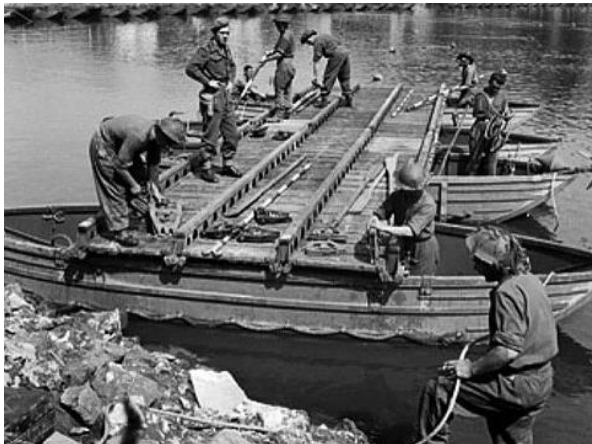
Folding Boat Equipment – FBE mk III
