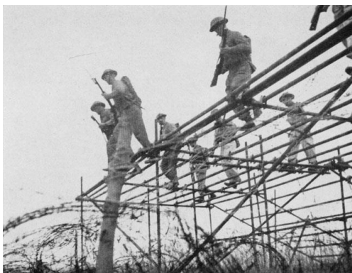
Scaffolding stage may have looked like this
