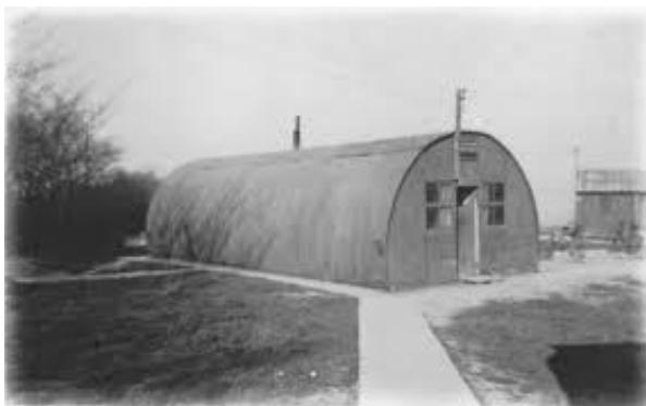
Erected Nissen Hut
