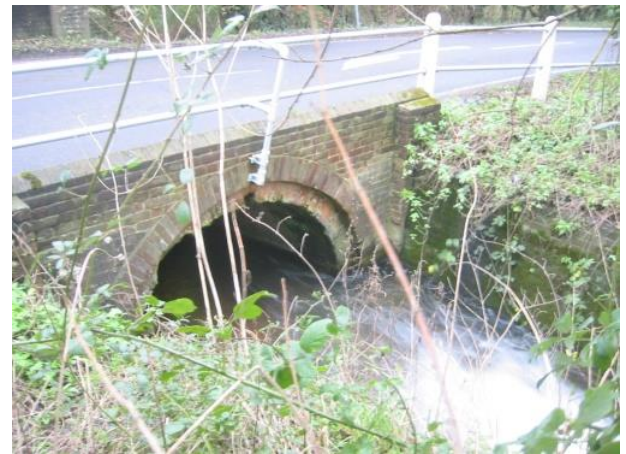
The Culvert under Emsworth Common Road
