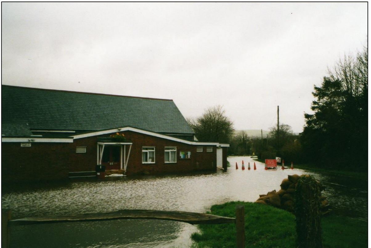
Figure 12 - 2000 The village hall and Pook Lane looking north.
