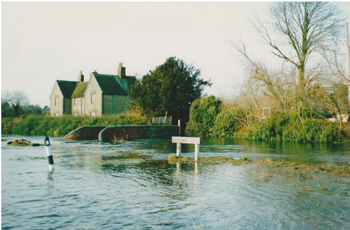
Figure 6 - Properties in Sheepwash Lane. The normal flow of the river restricted by the bridges and thus overtopping of the bank occurred.
