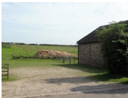
NW Entrance from Pook Lane
