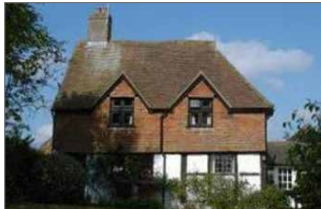
Figure 12B: Example of tile hung example of a timber frame building with dormer windows into the roof line
