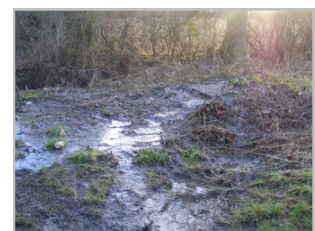
Overflowing sewer chamber on farmland west of Newpound Lane
