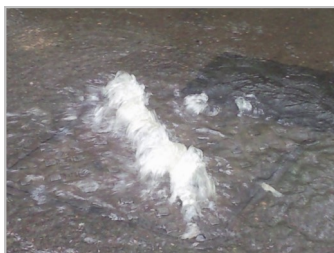
Overflowing sewer chamber in road in Newpound Lane
