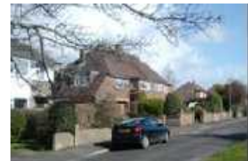
Lansdowne Road / Mill Road
