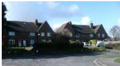
Palmer Road / Arundel Road
