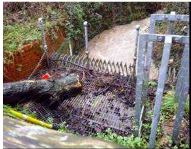
Figure 3.4: Black Ditch Culvert – Feb 2014
