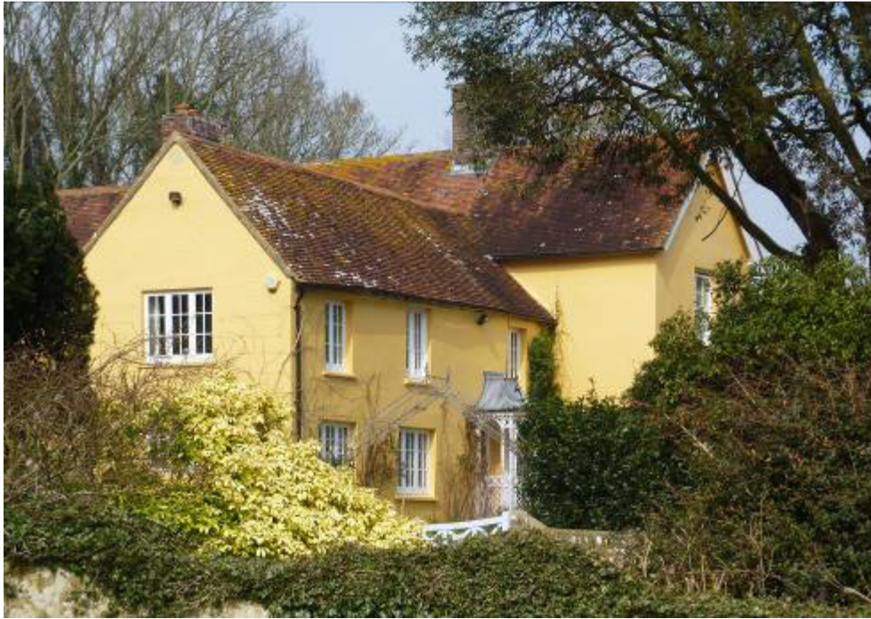
Figure 11: The Rectory: The south wing is a 16 th century timber-framed building refaced with stucco and bearing the date 1604. The east-west wing at its northern end is a 19 th century addition
