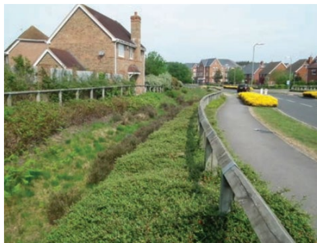
Figure 50: An example of a SuDS corridor - (Source: https://hydro-int.com/sites/default/files/hydro-brake-optimum-case-study-elvetham-en-gb.pdf )
