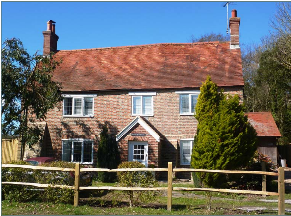
Figure 13: 18 th Century Grade II listed cottages. 14 Arundel Road (above) 12 Arundel Road, ( below)
