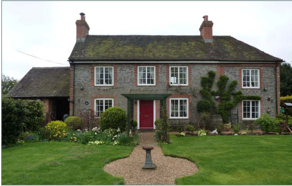
Figure 14: 18 th century Grade II listed cottage, 13 Arundel Road, Castle Goring Cottages (above) Cottage forming part of the second stable block, built c.1875 (below)
