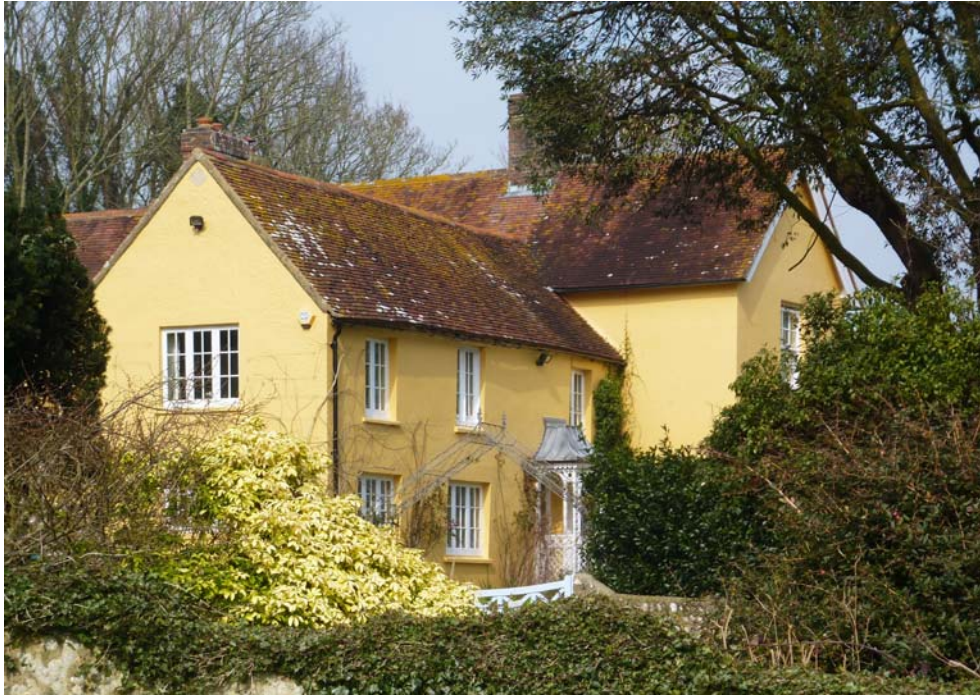
Figure 11: The Rectory: The south wing is a 16 th century timber-framed building refaced with stucco and bearing the date 1604. The east-west wing at its northern end is a 19 th century addition.
