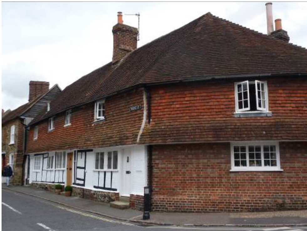
A timber-framed building, with continuous jetty, clad with vertically hung tiles
