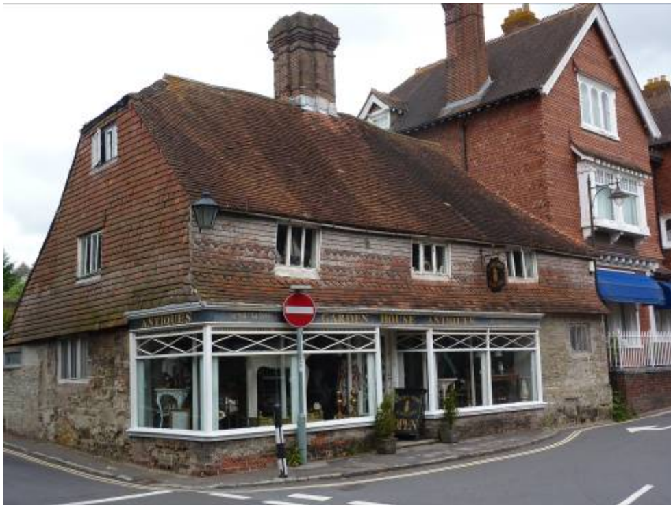
Timber-frame, masked by vertical tile hanging, over a greensand plinth
