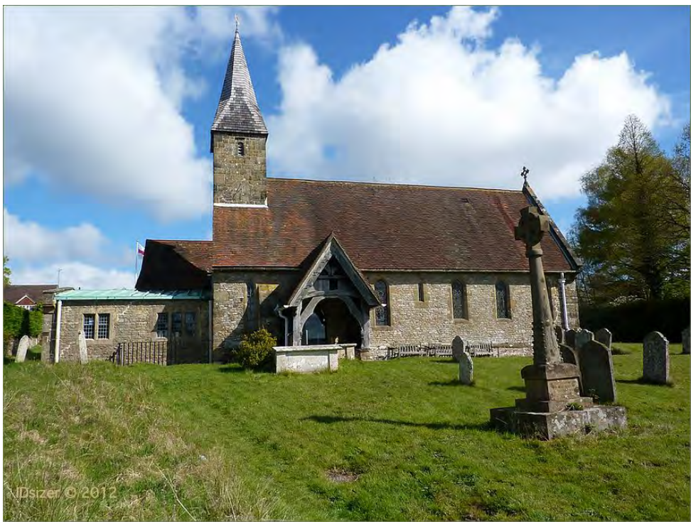
Figure 10: South face of the Church seen from Churchyard
