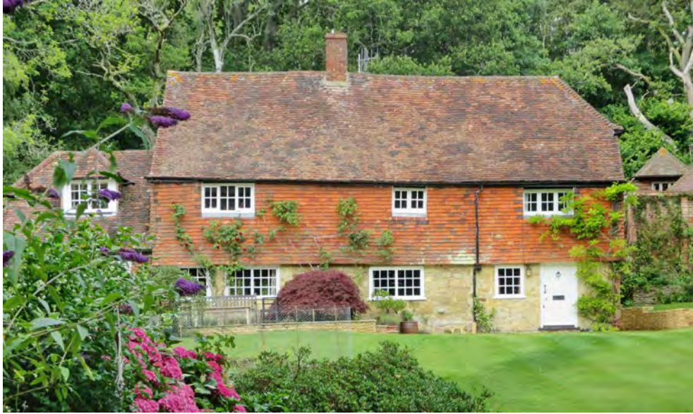
Figure 20: Many of the scatter of houses to each side of the road to Shulbrede, such as Waterhouse Cottage are datable to the Sixteenth and Seventeenth Centuries and may incorporate materials from the former Priory
