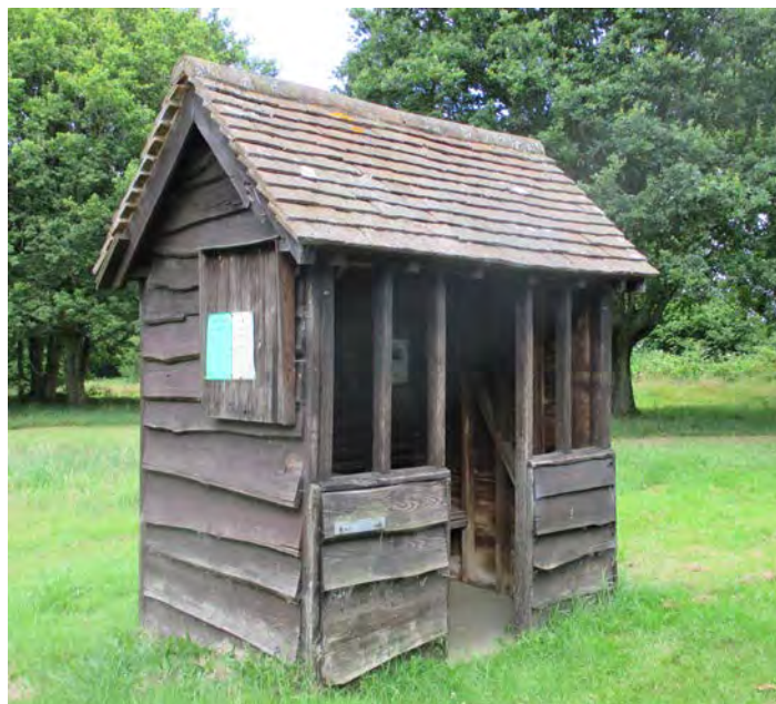
Figure 14: Bus Shelter on the Green
