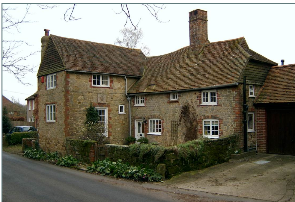
Park View, Church Lane – Greensand rubble with brick dressings
