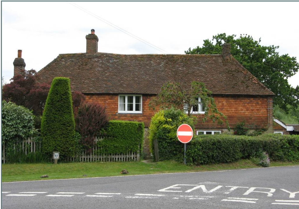
Clay plain tiles, used for both roofs and as a cladding are a characteristic of Wealden vernacular buildings
