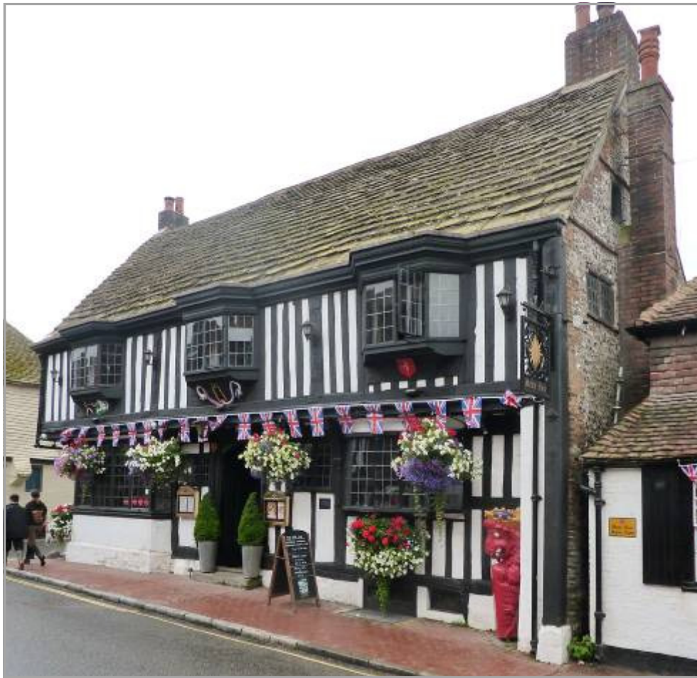
Figure 22: The Star Inn (Grade II* listed) is a good example of a 15 th century timber-framed building. The closely spaced vertical timbers are called “studs” and when they are placed close to each other as on this building, it is called “close-studding”. The gaps between the studs are filled with plaster. The first floor projects over the ground floor supported by a large timber beam called a “bressumer”. This has carvings, including that of St George and the Dragon shown below.
