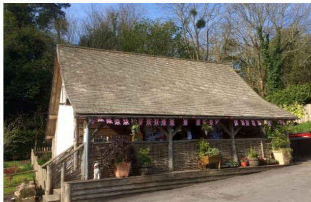
Roof of Lodsworth Larder (see 9.3)
