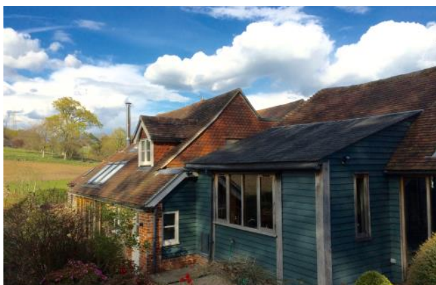
Mix of tiles and slate on extensions to stone cottage and timber framed barn (see 9.6 and 9.7)
