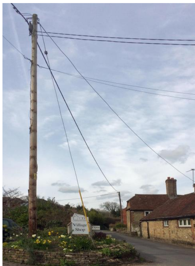
Existing very prominent overhead cables (see 9.9)
