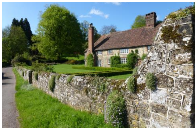
Stone wall between highway and garden (see 7.5)
