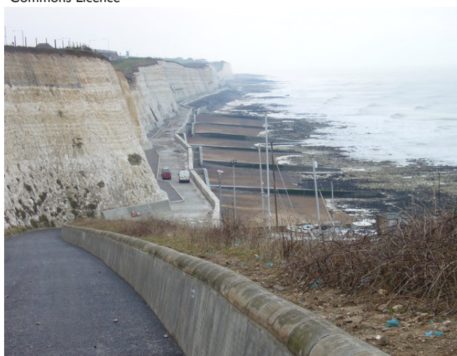
The Undercliff Walk, providing easy access along the base of the cliff and acting as a sea defence.
