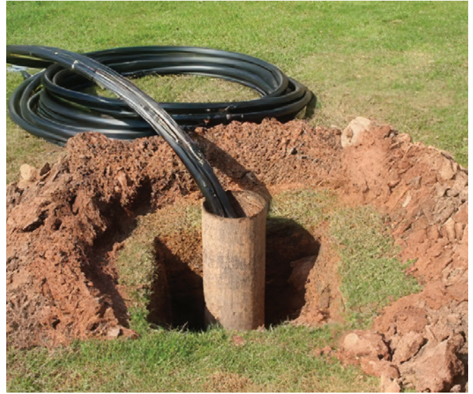
FIGURE 21: EXAMPLE OF A BORE HOLE (HISTORIC ENGLAND)
