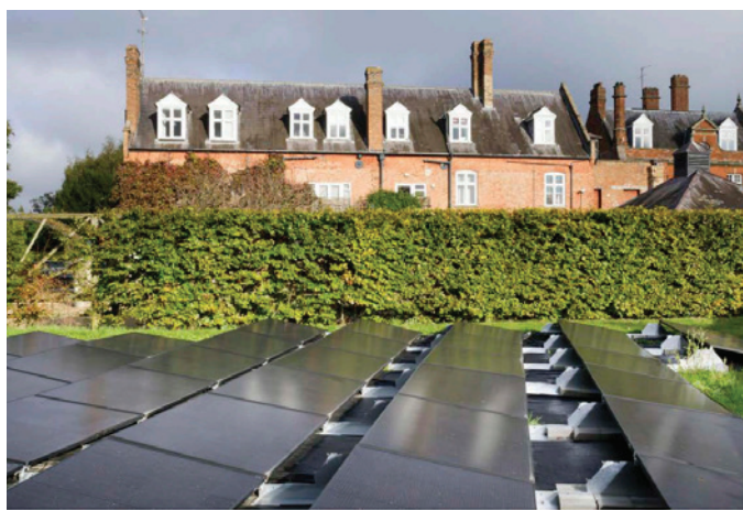
FIGURE 16: GROUND MOUNTED SOLAR PANELS IN A GARDEN (HE ADAPTING HISTORIC BUILDINGS FOR ENERGY & CARBON EFFICIENCY 2024)
