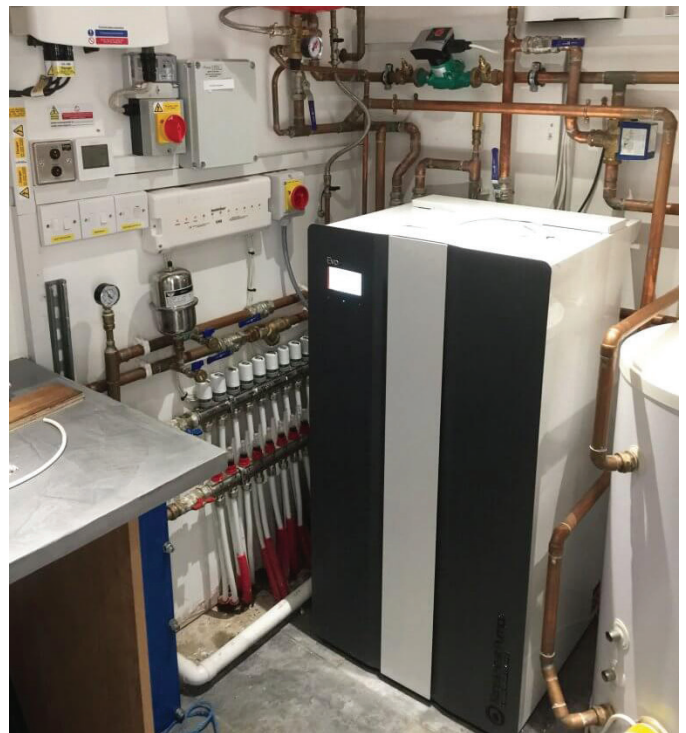
FIGURE 22: TYPICAL PLANT FOR DOMESTIC HEAT PUMP (SELF BUILD)
