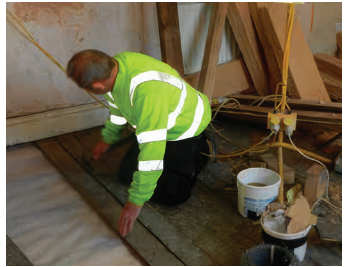
FIGURE 4: INSULATION WITHIN THE FLOOR.
