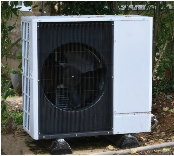
FIGURE 18: A TYPICAL DOMESTIC-SCALE AIR SOURCE HEAT PUMP (SELFBUILD.UK)
