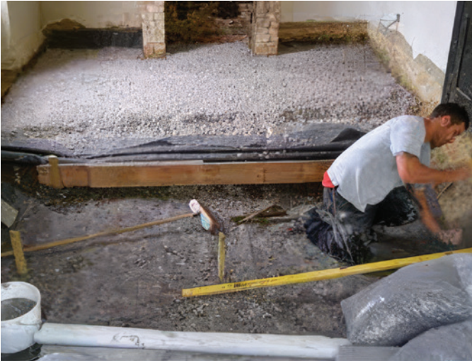
FIGURE 5: AN INSULATED HYDRAULIC LIME FLOOR BEING LAID.
