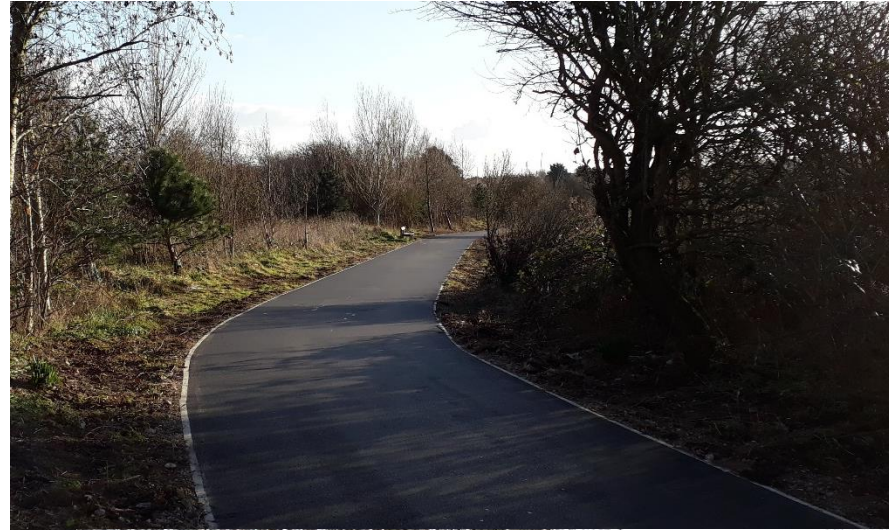
Opened February 2022 Re-profiled, widened to 3m, sealed surface and concrete edging.
