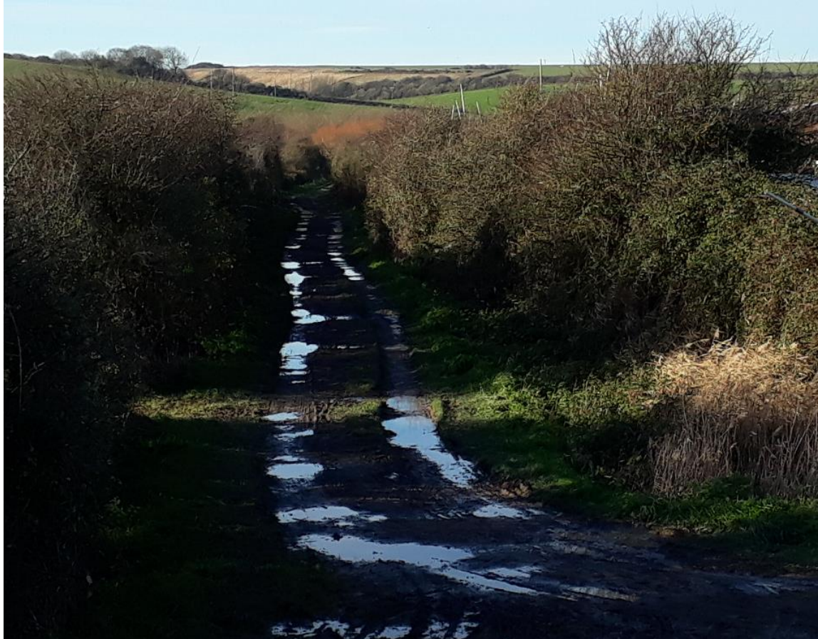
Newhaven and Seaford Sailing Club (NSSC) access track (approx Chainage 920-650) looking west
