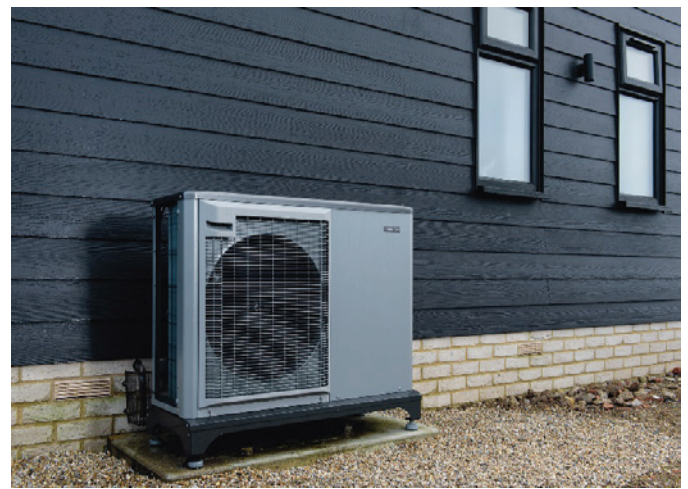
FIGURE 16: A TYPICAL DOMESTIC-SCALE AIR SOURCE HEAT PUMP (SELFBUILD.UK)
