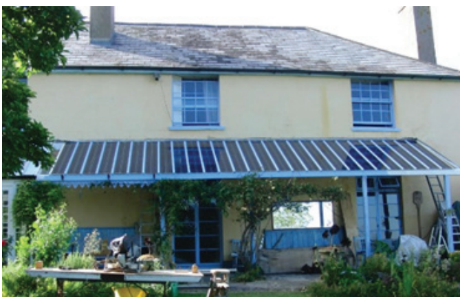
FIGURE 14 (LEFT): SOLAR PANELS IN A DISCREET LOCATION ON LEAN-TO
