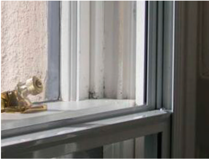
FIGURE 11: SECONDARY GLAZING (HISTORIC ENGLAND (2024) ADAPTING HISTORIC BUILDING'S FOR ENERGY AND CARBON EFFICIENCY)
