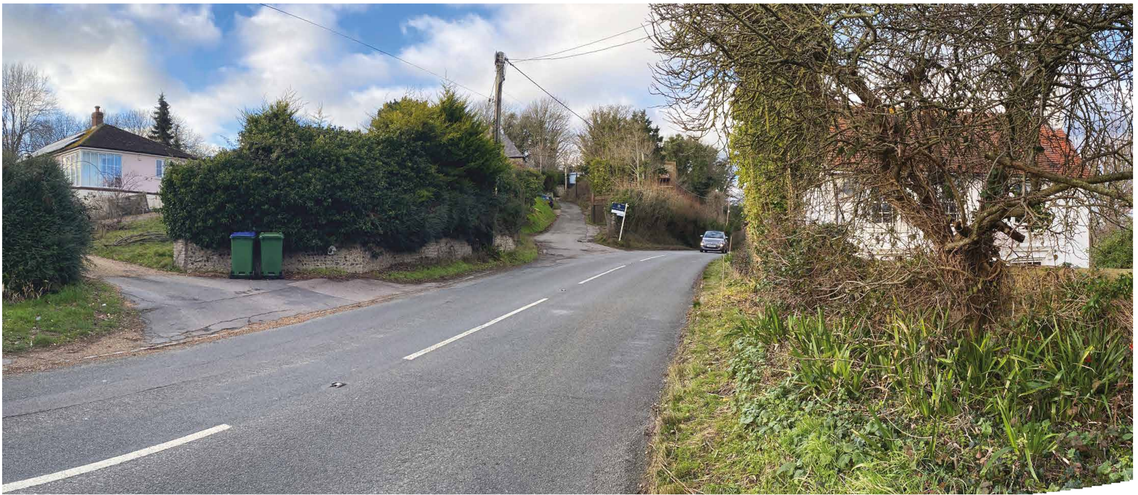
Location 2 - Existing View North of The Street looking towards Harping Hill
