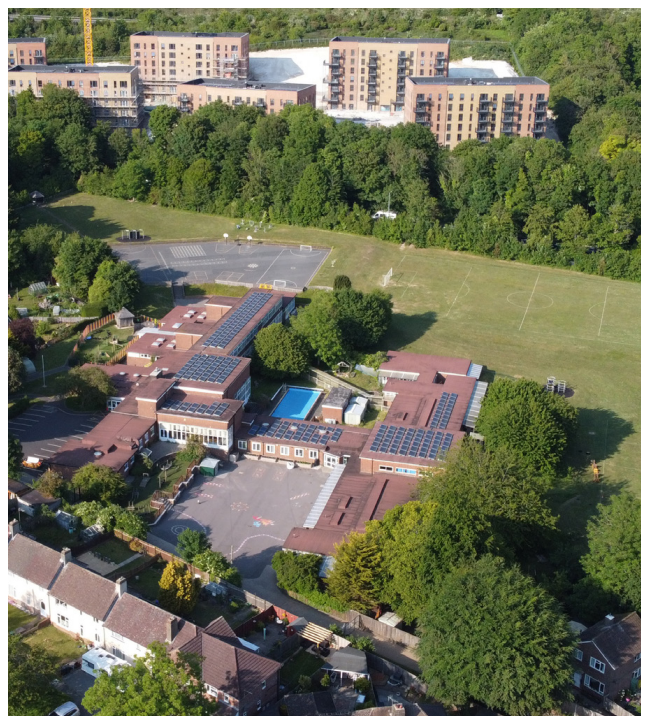
Figure 9: Coldean Primary School and Bluebell Heights Development
