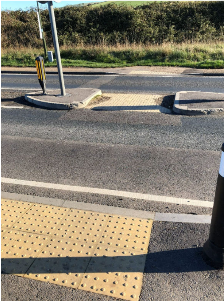
Figure 18 - Pedestrian Refuge Island of A283
