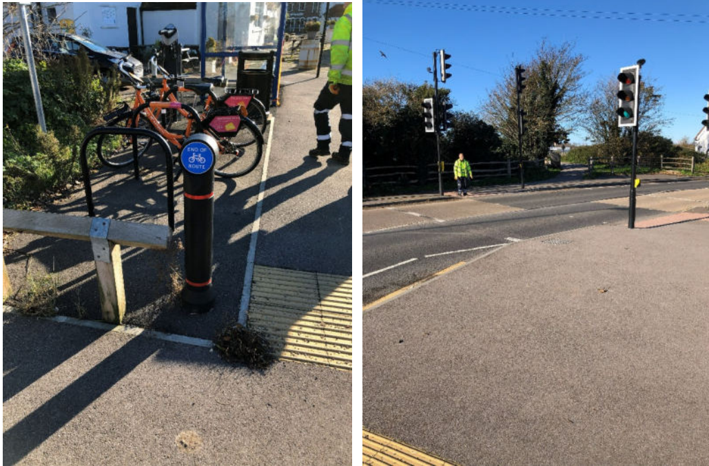
Figure 26 - Southern Terminus of Downs Link
