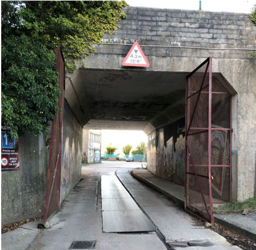
Figure 2 - Underpass Access Route
