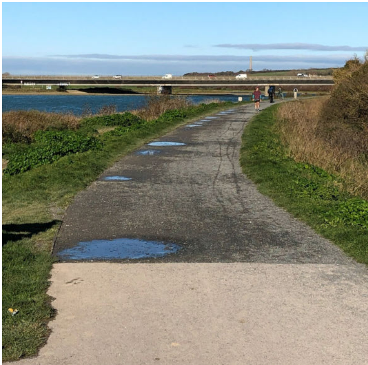
Figure 22 - Change in Downs Link Surface Finish - Asphalt to Compacted Gravel
