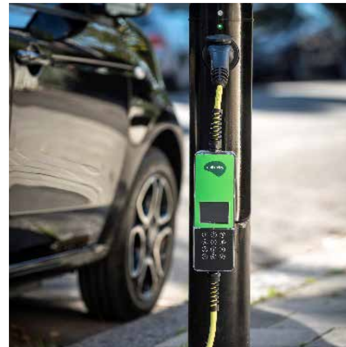
Fig. 8.26: A converted lamp post housing an on street EV charge point (Lucy Zodion)
