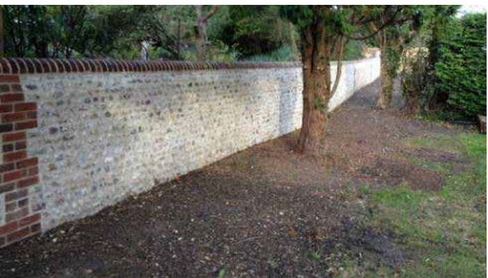
Fig 12.9: A well built, new flint wall with masonry piers and coping
