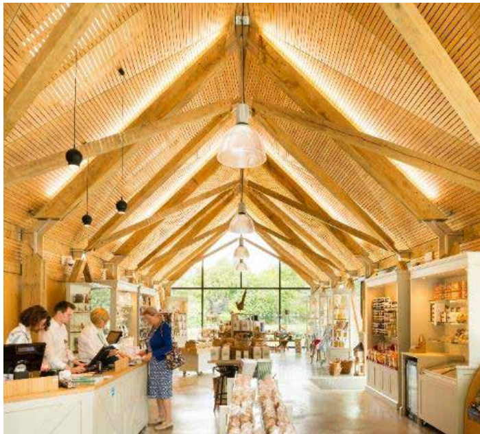
Figs 12.23: Locally sourced oak timber frame
