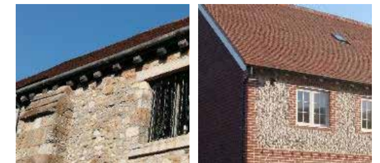
Fig 13.14: Exposed rafter feet with eaves ventilation between them on medieval building in Southampton and in a new development in East Dean (BETTER PHOTO)
