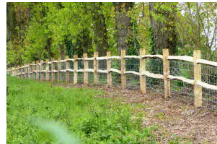
Fig 12.36: Chestnut cleft post and rail fencing with wire mesh animal proof fencing attached.
