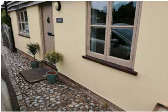
Fig 12.22: House in Hambledon showing how render is protected from ground splash back with brick detail
