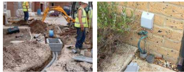
Fig 8.18: a) Laying ducting (BT Openreach) with inspection chamber and b) duct end with drawstring to allow for future easy laying of fibre cable to a house.
