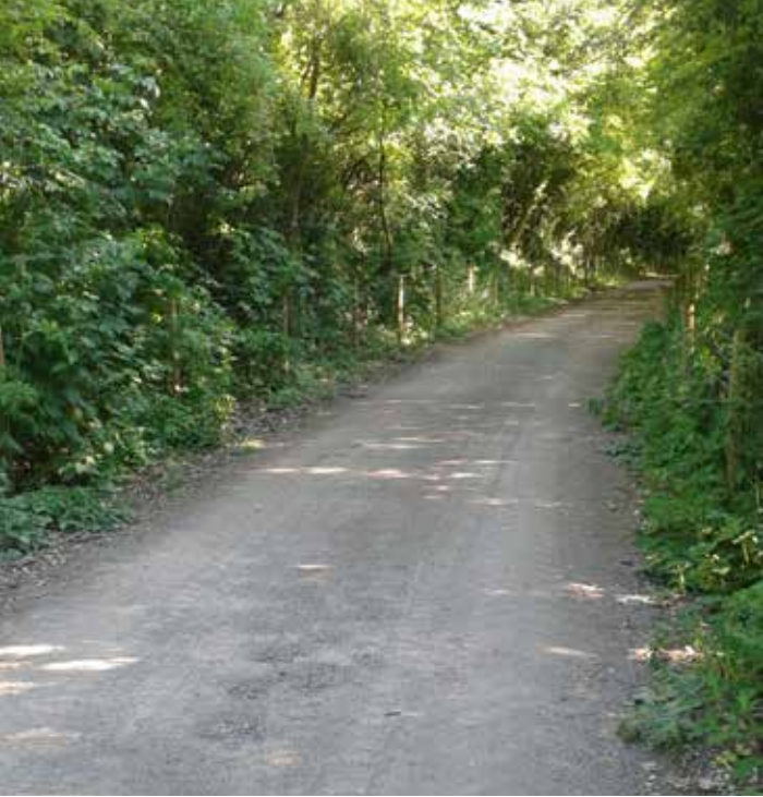
Fig 12.40: Centurian Way (between Chichester and West Dean) is a good example of a rural cycle (and pedestrian) route with a very simple construction using local materials. (A self-binding limestone dust over a 'Type 1' graded stone sub-base with no edge details or kerbs).
