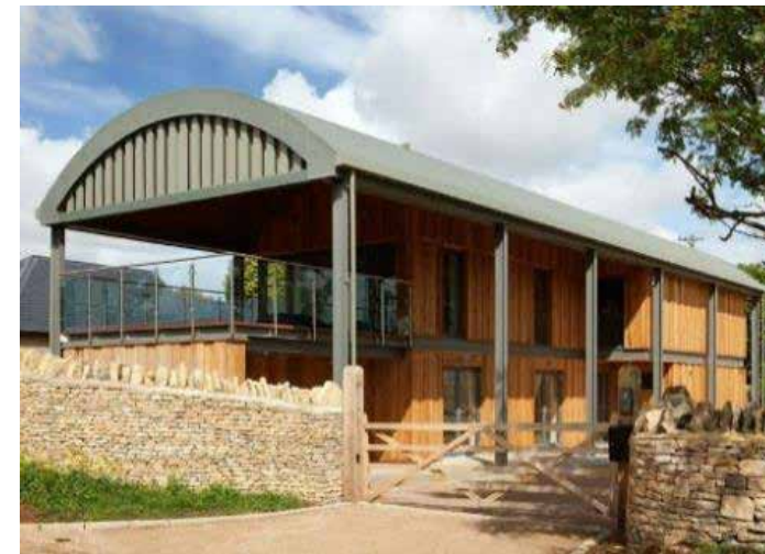
Fig 5.5: Successful conversion of steel framed open cattle shed in Devon
