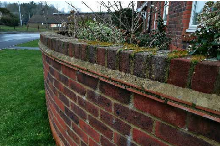
Fig 12.8: Traditional tile creasing in brick wall coping detail, in modern Midhurst development
