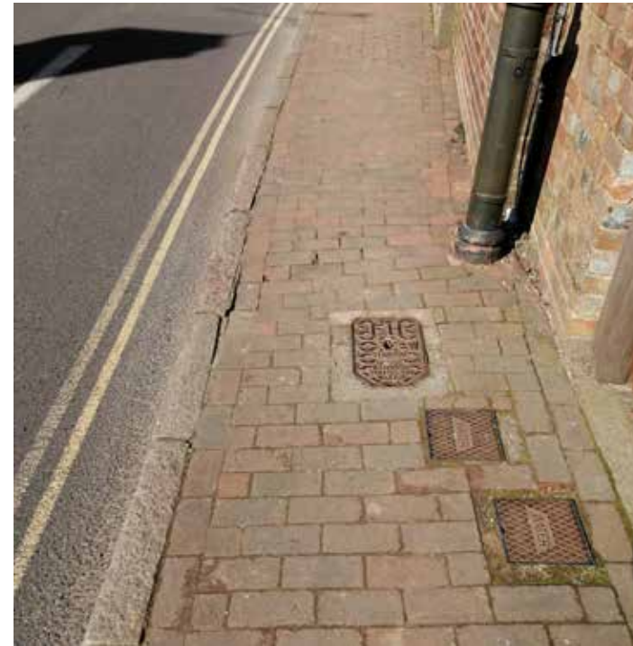
Fig 12.44: Concrete block pavers (here 'Tegula' in Petworth) are widely used in more urban contexts. This can lead to an 'anywhere' character whereas local stone or clay pavers are preferable as they reinforce local character.
