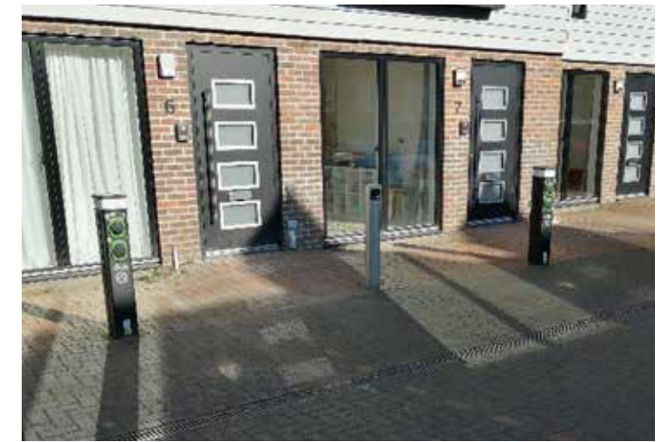
Fig. 8.27: EV charge points serving residents in a flatted development in Lewes and also serving as traffic bollards
