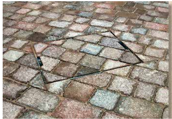
Fig 8.16: Service manhole recessed cover helps to protect integrity of paving, even when at an angle. (Pavingexpert.com)
