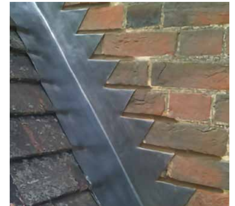
Fig 12.29: Good quality flashings in a roof junction
