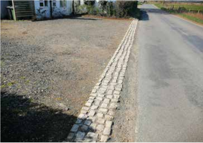
Fig 12.37: Courses of granite setts create an appropriate and robust edge between a rural road and a private, stone-surfaced drive, near Owlesbury
