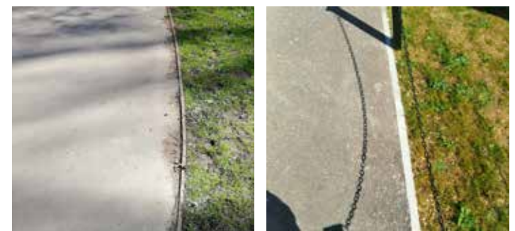
Fig 12.49: Timber edge detailing (Midhurst, left) has a more low-key visual impact than concrete pin kerbs (Cheriton, right). Timber can be more appropriate in rural contexts or where a more 'natural' approach is called for.
