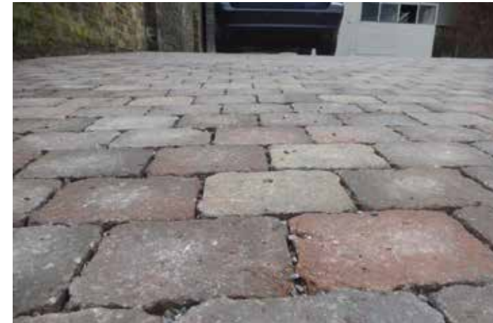
Fig 12.46: Permeable block paving on a private drive is designed with nibs to keep gaps between blocks open to allow water infiltration.
