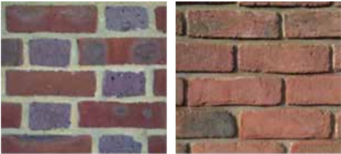
Fig 12.5: Mortar coursing has a profound effect on the appearance of brickwork
