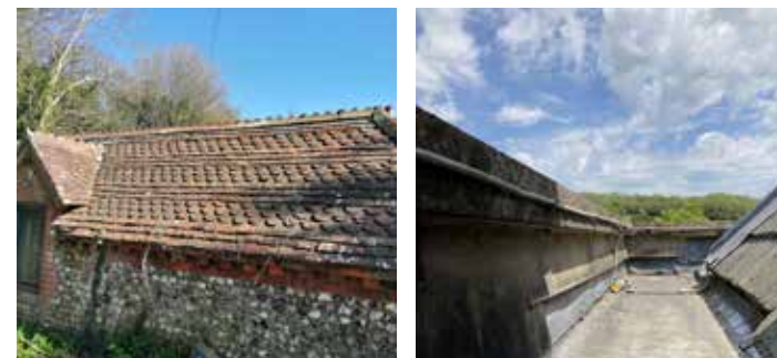
Figs 13.11 and 13.12: Traditional roof ridge detail and parapet and secret gutter
