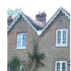
Centre valley gutters are found on many houses in Liss, either transverse or parallel to the front of the house. If they are to be emulated, then the valley must be carefully designed for regular maintenance and preventing the hopperheads from icing up when the snow in the valley starts the process of melt and freeze
